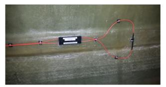
Fig. 2.14 Cable fixed with plastic clamps
