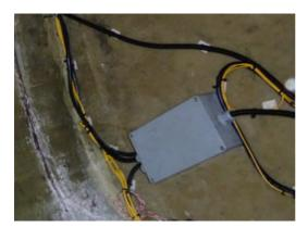
Fig. 2.16 Protection boxes for extra cable and connections
