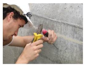
Fig. 2.1 Removing irregularities of the surface
