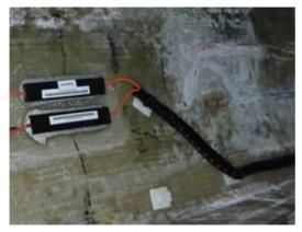
Fig. 2.15 Cable protected with corrugated tubes
