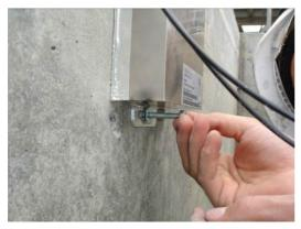
Fig. 2.5 Applying the washers and hexagon nuts
